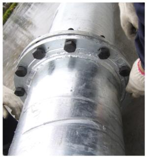
2. To connect the steel wire after connecting the tower as below picture. For safety, you could twine the tower with the steel wire for a circle before fixing the wire with the fixture. There need to be two fixtures for each steel wire, and 10-20 cm need to be left in the end of the wire
