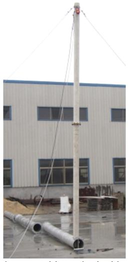
Aim the pin hole of tower to the basement, and insert the pin with smearing grease, as below
