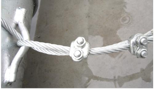
Besides aiming the steel wire for front basement, the ends of all other steel wire need to connect with the corresponding basement. And you could fix all wires after the installation of the tower as below
