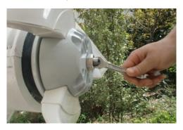
6. Install the nose cone onto the generator;
